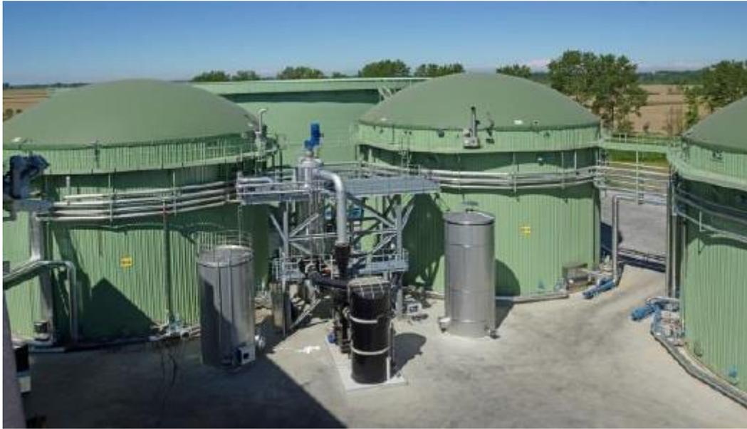
Picture 2 Anaerobic Digestion tanks
