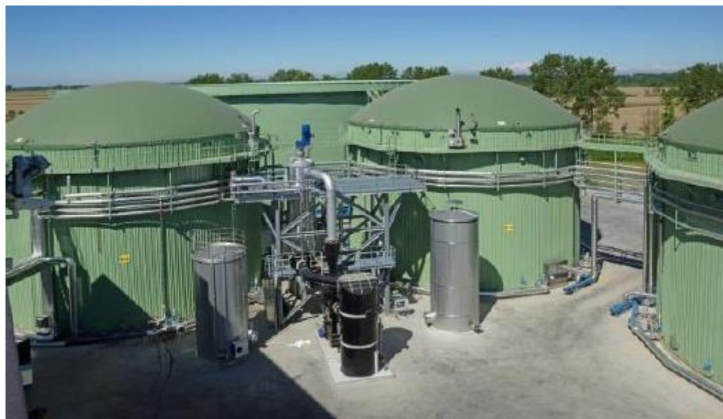
Picture 2 Anaerobic Digestion tanks
